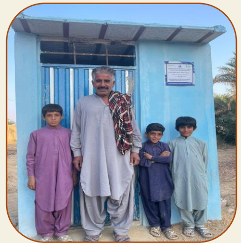
Completed latrine (post-construction)
